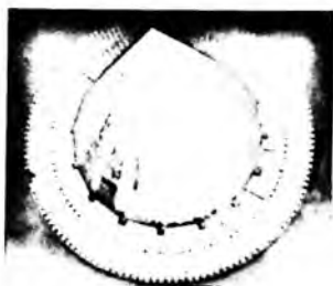
161 – rasm. Sement silosining tubidagi konus ko'rinishi [153]
