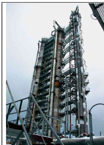
11.14 -rasm. Chapdan o‘ngga: tovar propilenini olish kolonnasi, tovar etileni olish kolonnasi
