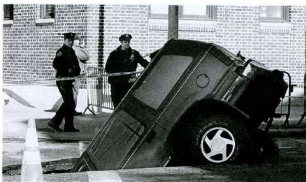
A car falls into a sinkhole
