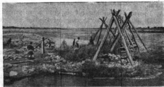
1.8 - rasm. Daryo o'zaniga sepoya o'rnatish.
