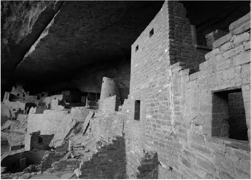
FIGURE 16. Dated to between 1190 and 1260 CE, and abandoned by 1300, Cliff Palace, like many Ancestral Pueblo settlements of the period, was constructed with towers situated within massive rock alcoves. Photograph © 2017 Rubén G. Mendoza.
