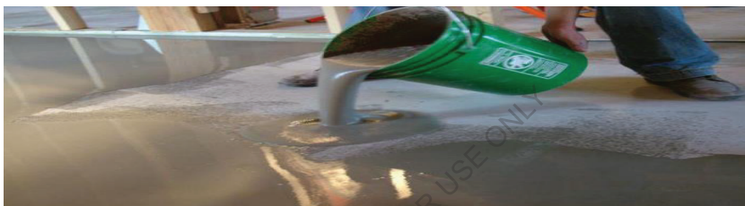
48-rasm. Polimer betondan pol quyish jarayoni
