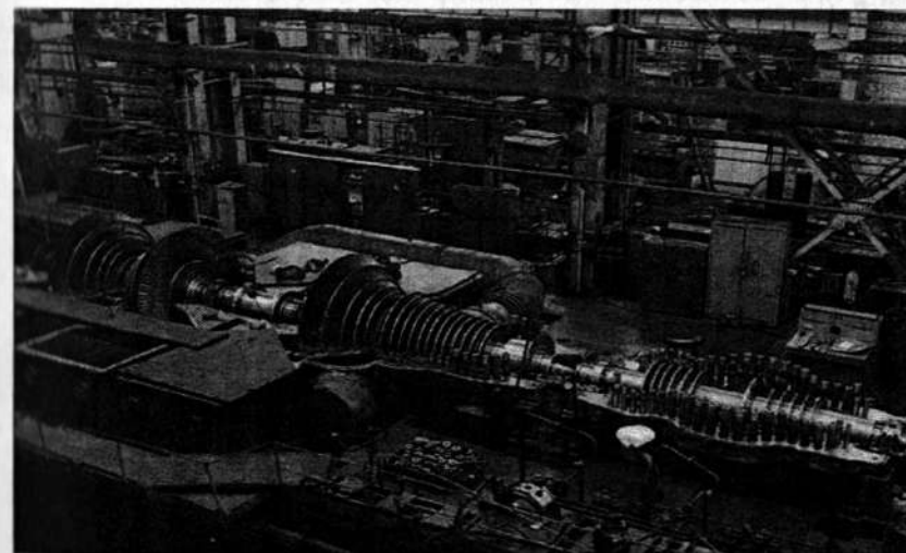
T-250/300-240 turbinaning tuzilishi (quvvati 250/300; bug'ning kirish bosimi -240 atm(kg/sm 2 )).
