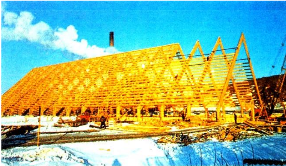
13.9-rasm. Arkalarni joyiga o'rnatish jarayoni
